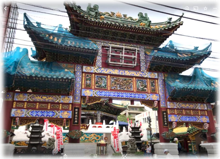
Archway (before renovation)
