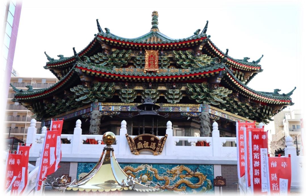
Main hall (before reconstruction project)
